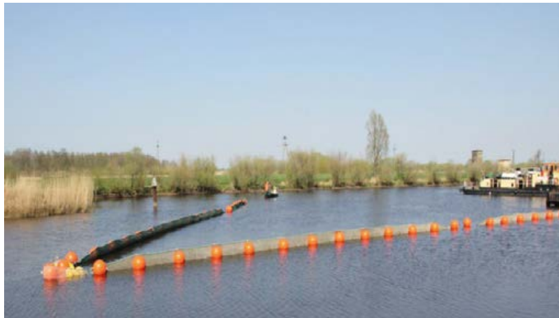
Figure 9: The boom in operation
